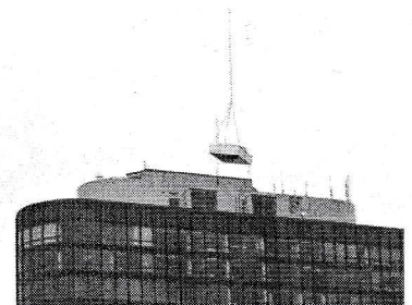
Cooling Tower landing safely
