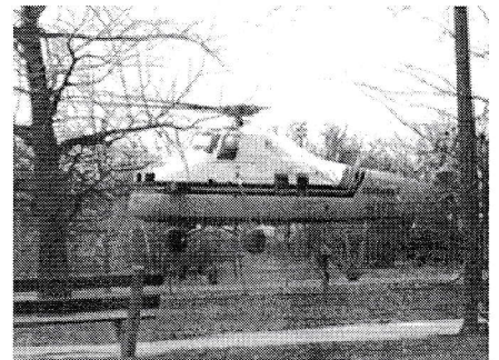
Lift Off for Cooling Tower Replacement Project on April 4, 2008
