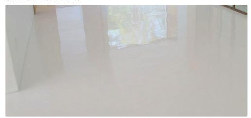
The solution, "Hermetic Neat Floor," is created by pouring, then rolling, successive layers of self-leveling liquid epoxy onto a solid subfloor, followed by a coat of protective urethane.
