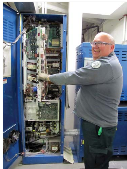
Brad Gibbs, Otis technician, at the controls of a hi-rise (gearless) elevator. Photo by Mike Magliane.
