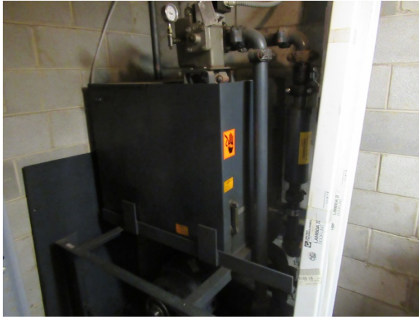
Power unit housing for the refuse elevator
