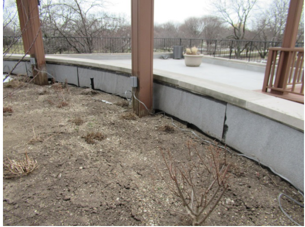
Recently replaced planter at 2 nd floor roof
