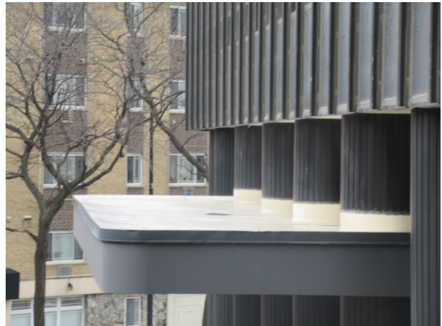
Roof membrane at lobby canopy
