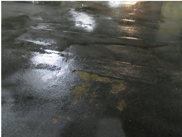
Traffic coating deterioration/damage at elevated garage floor
