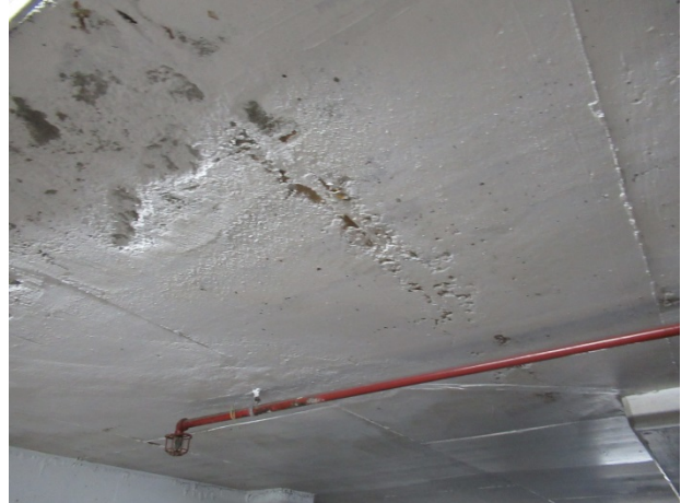
Typical concrete repairs beneath elevated garage floor
