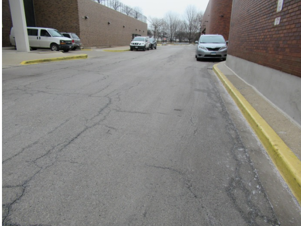
Pavement deterioration at north perimeter
