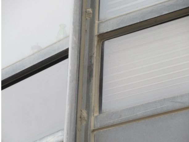
Sealant at metal/glass and metal/metal interfaces
