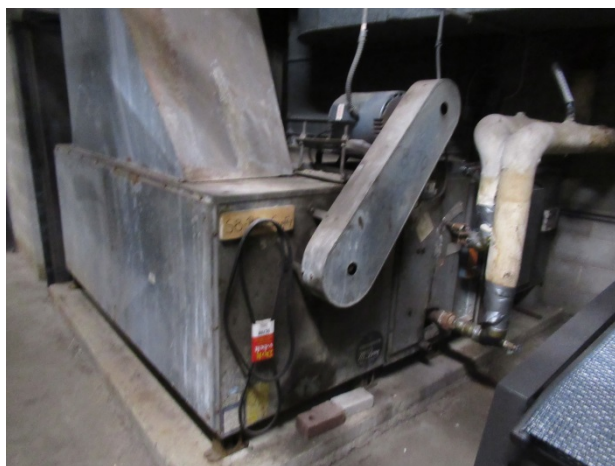
Pool air handling unit
