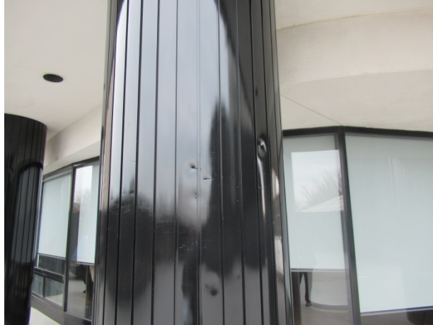
Damage at column cladding
