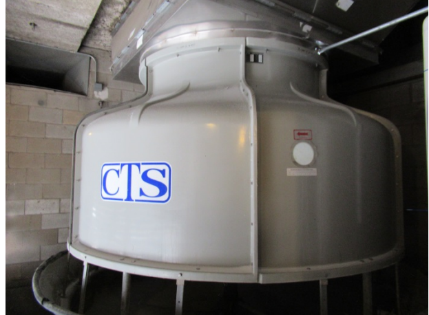
Commercial cooling tower
