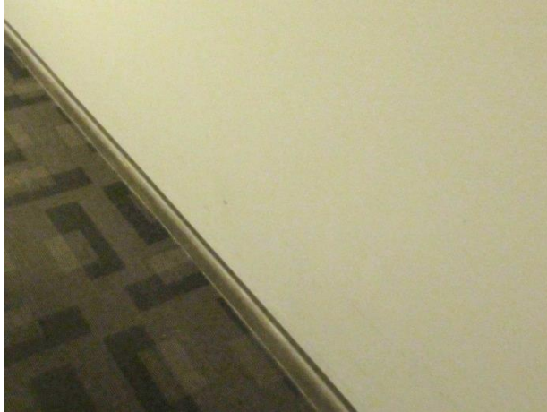
Typical scuff at hallway wall
