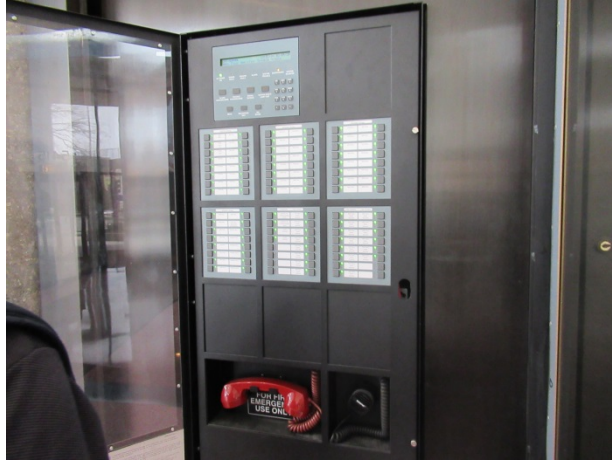
Central control panel
