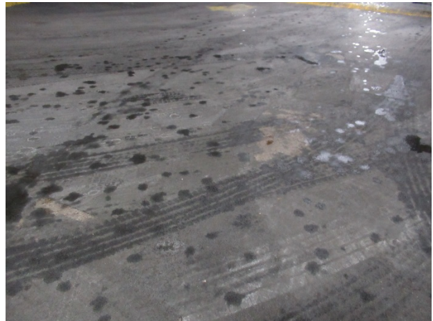
Traffic coating deterioration/damage at elevated garage floor
