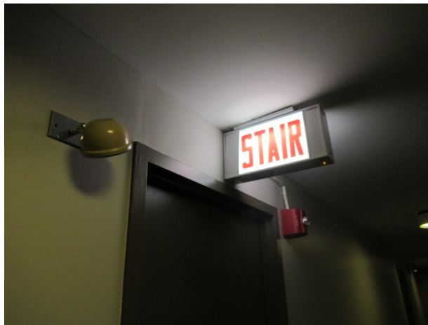
Fixtures at hallway
