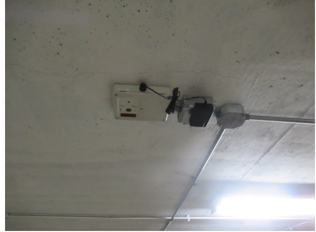
Garage CO detector
