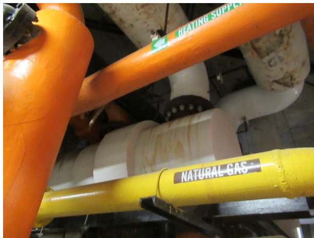
Heat exchanger for residential unit heat
