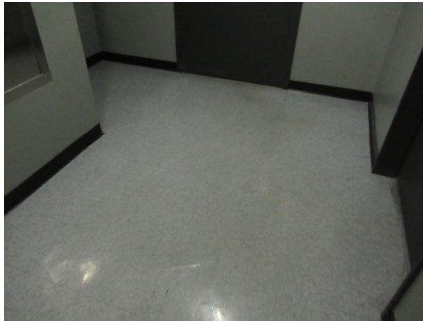
Flooring at service elevator foyer
