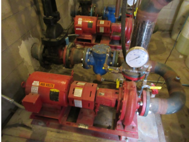
Pumps for commercial cooling system at cooling tower
