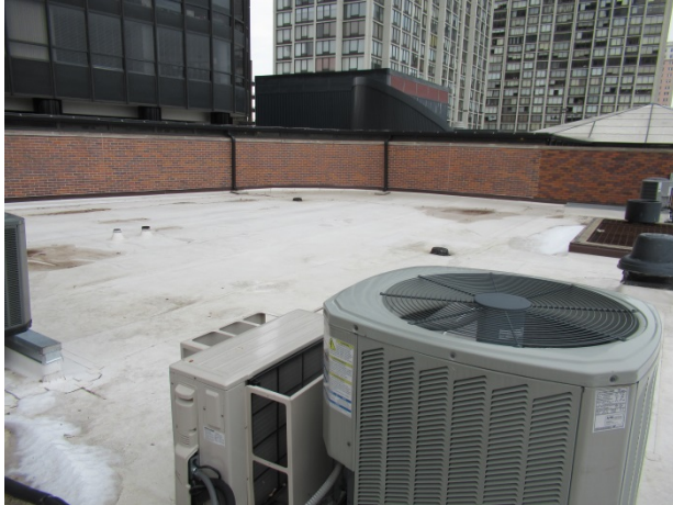
Roof system at 2 nd floor center/east
