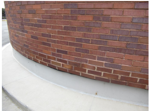
Masonry deterioration and lack of flashing at wall base
