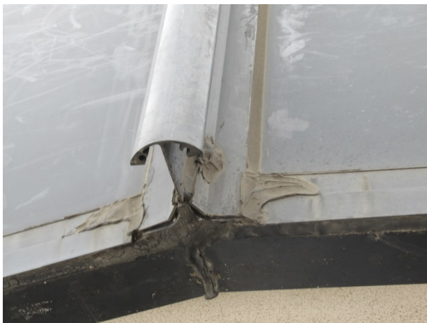
Sealants at base of vertical mullion
