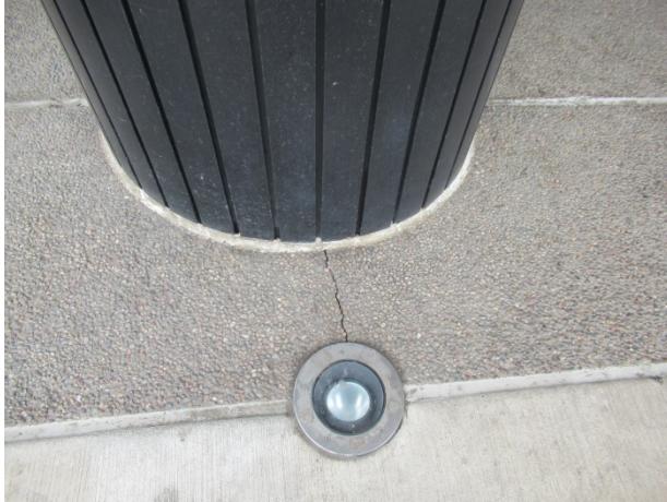
Crack in concrete plaza
