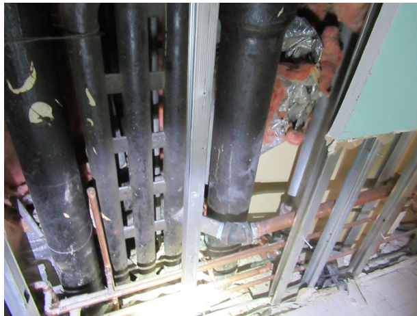
Domestic water system risers
