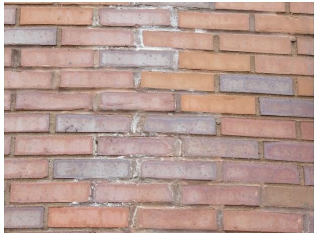
Evidence of water infiltration at masonry wall
