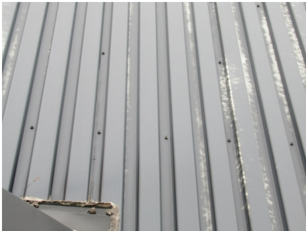
Metal siding finish damage
