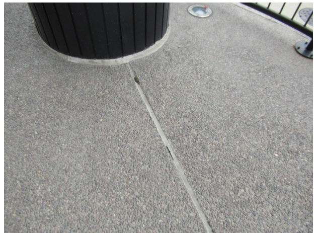
Sealant deterioration at plaza
