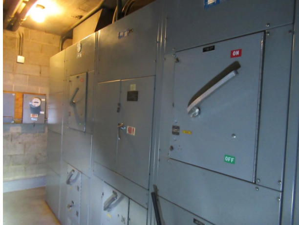
Electrical distribution panels
