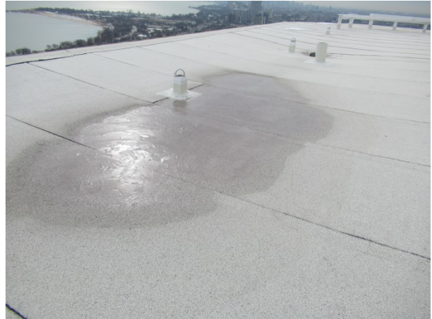
Lack of drainage at main level roof system
