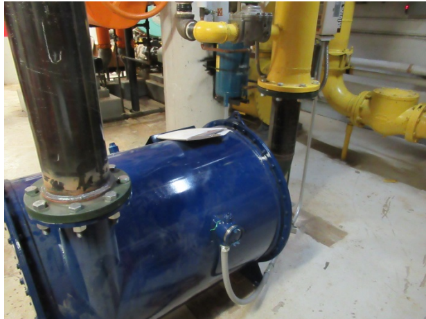
Gas booster pump
