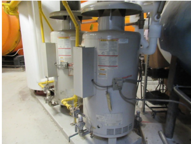
Commercial domestic water boilers
