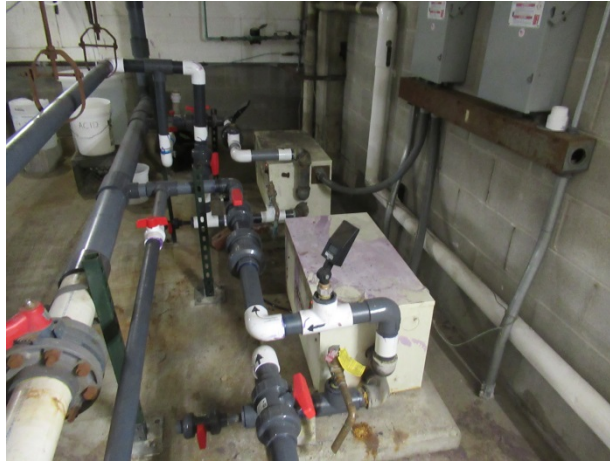
Pool mechanical equipment
