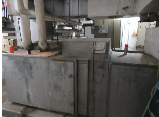
Basement level and party room air handling units
