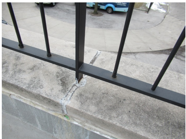
Inset post and steel rust at 2 nd floor roof perimeter
