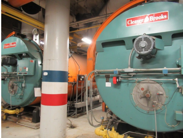
Building heat boilers
