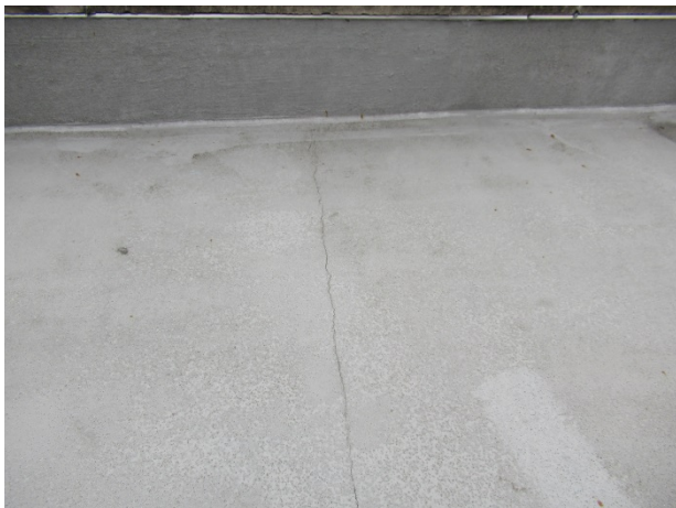
Crack at waterproof coating at 2 nd floor concrete roof system
