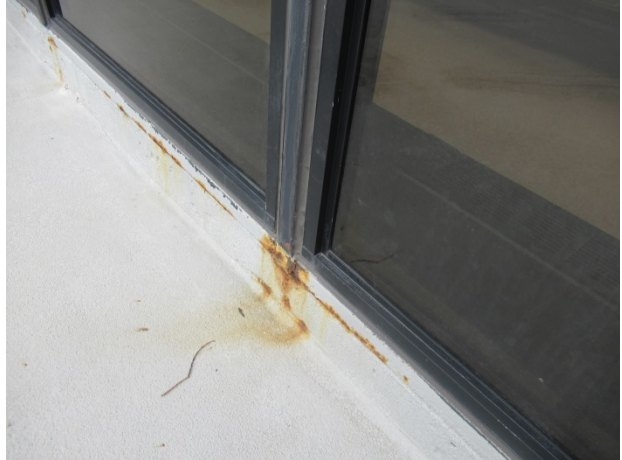
Window system at walkway to pool
