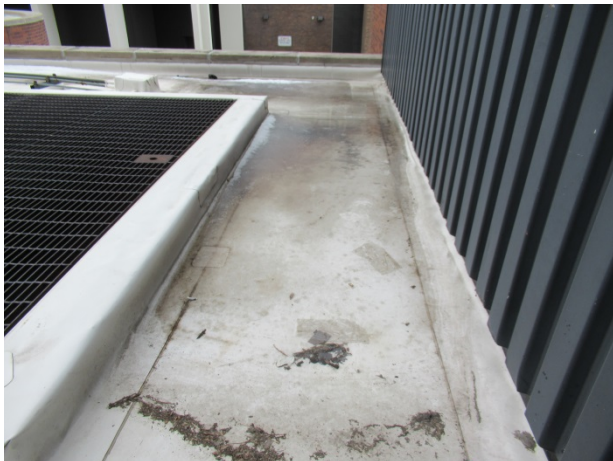
Lack of drainage at roof at 2 nd floor northwest
