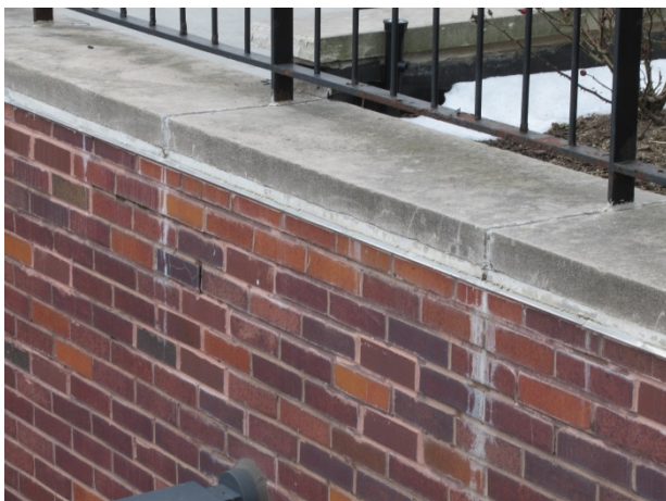
Evidence of water infiltration at masonry wall
