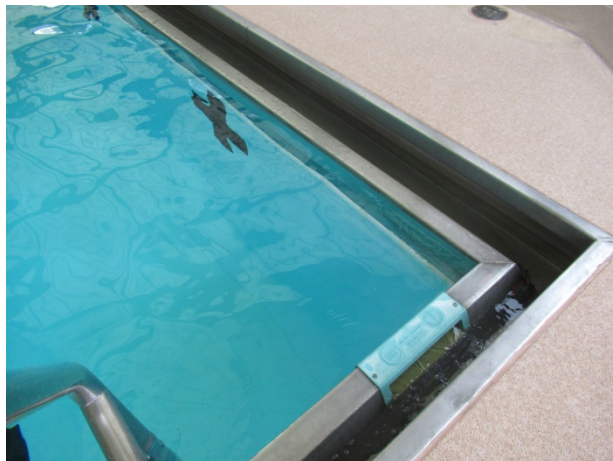
Liner at indoor pool
