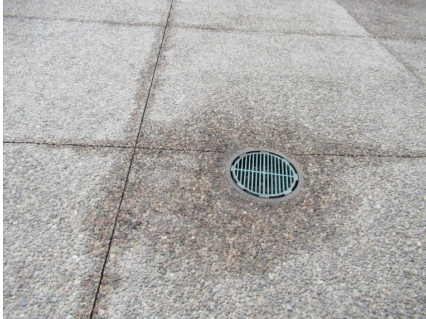
Plaza at drain
