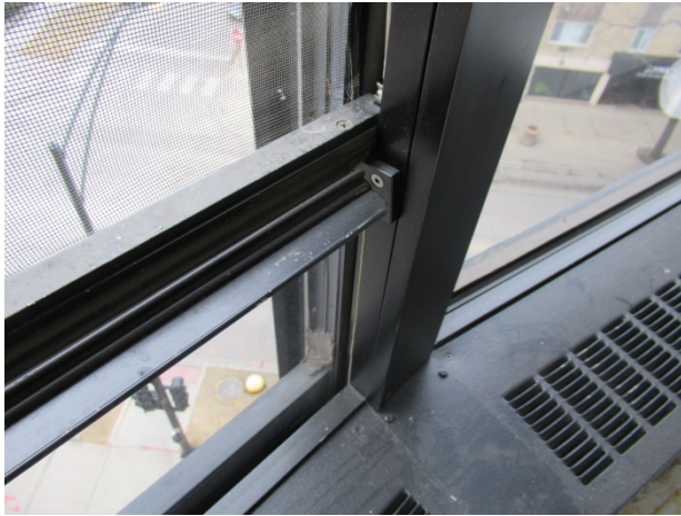
Residential unit curtain wall system at operable window
