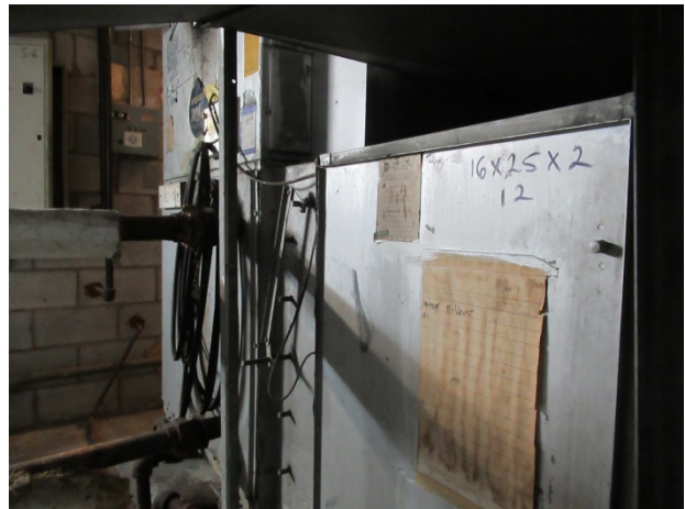
Mall air handling unit
