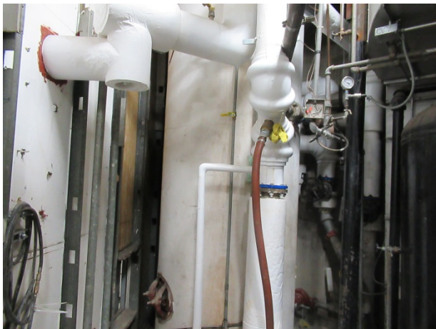
High zone domestic hot water storage tank
