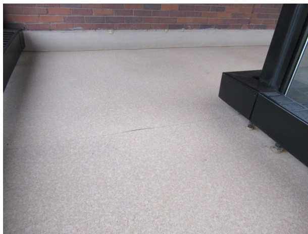
Raised seam at walkway flooring
