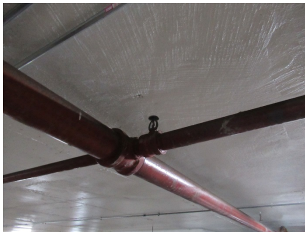
Fire suppression system pipes and head
