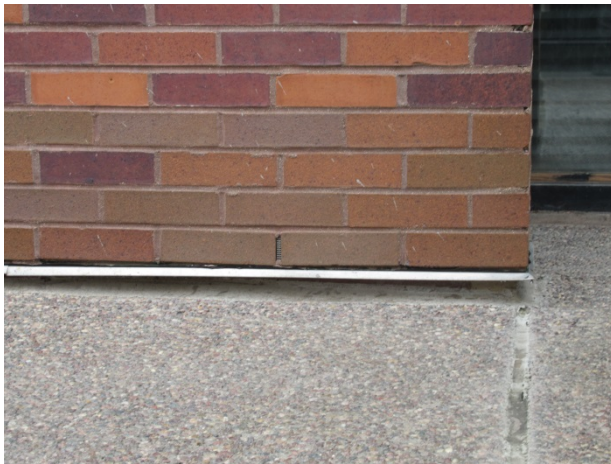
Flashing installed at base of masonry wall
