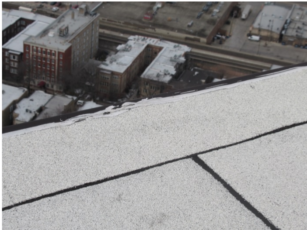
Perimeter sealant at main level roof
