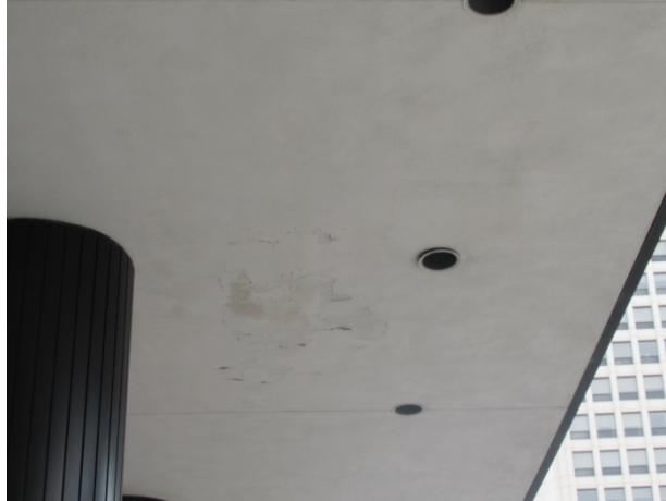
Soffit paint finish deterioration
