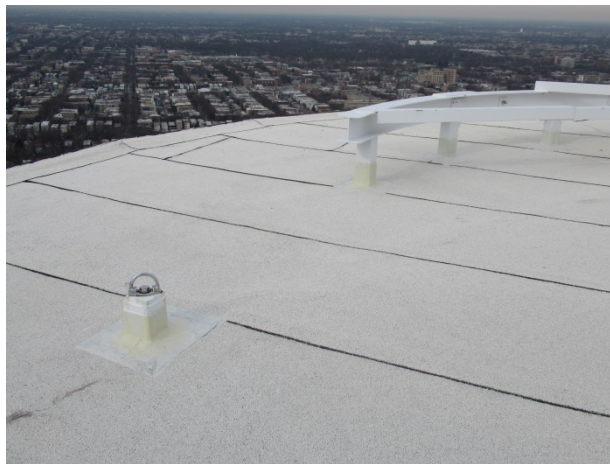
Roof anchor and original track system
