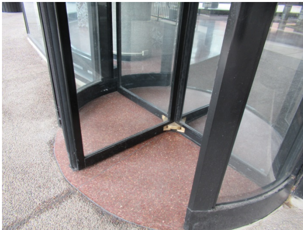
Lobby revolving door
