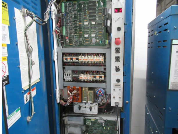
Traction elevator controls
