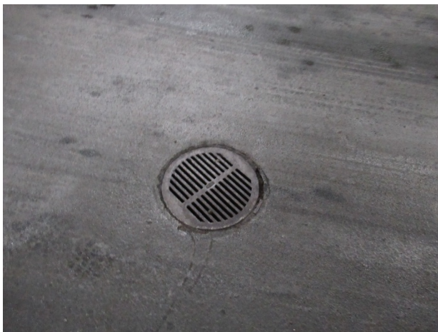
Traffic coating deterioration/damage at elevated garage floor at drain
