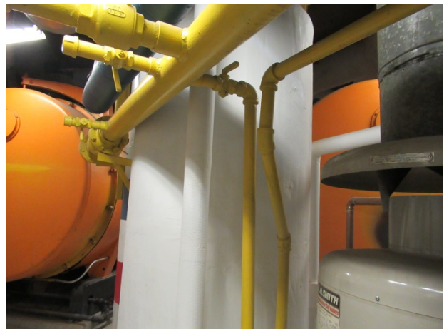
Recently installed storage tank at boiler room
