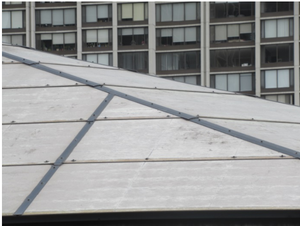
Pool enclosure roof system
