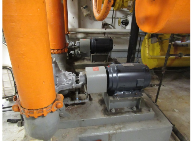
Pumps for commercial building heating system
