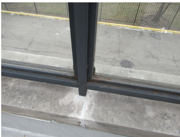
Frame corrosion at railing east of pool area
