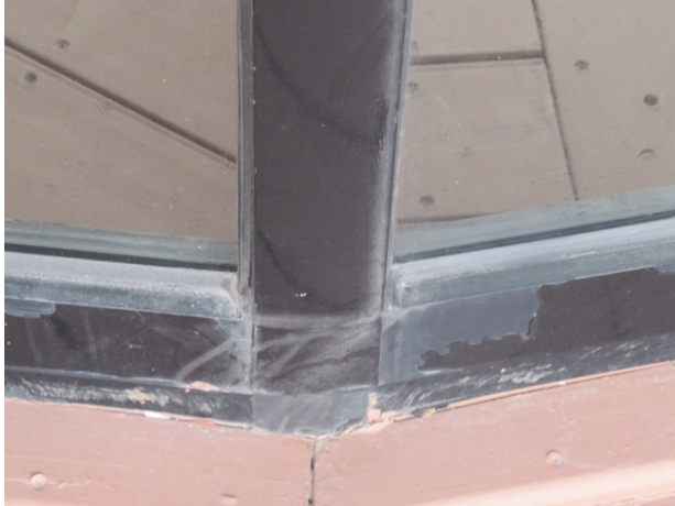
Window system at 2 nd floor at sun deck area
