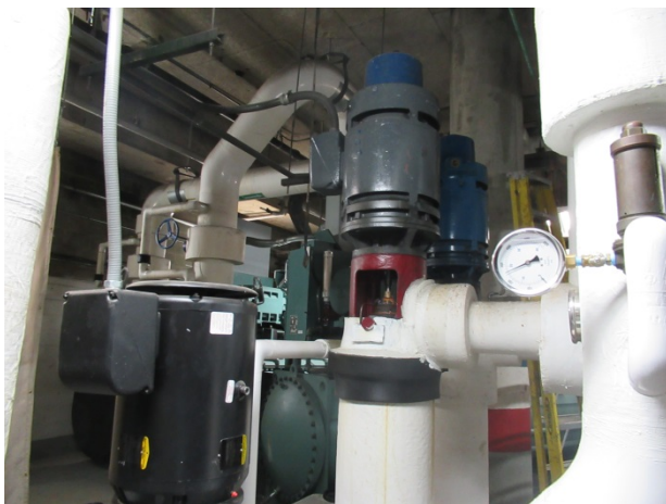
Domestic cold water pumps
