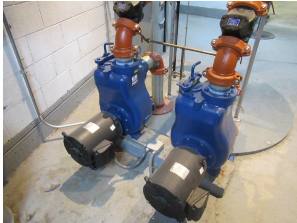
Sewage ejection pumps
