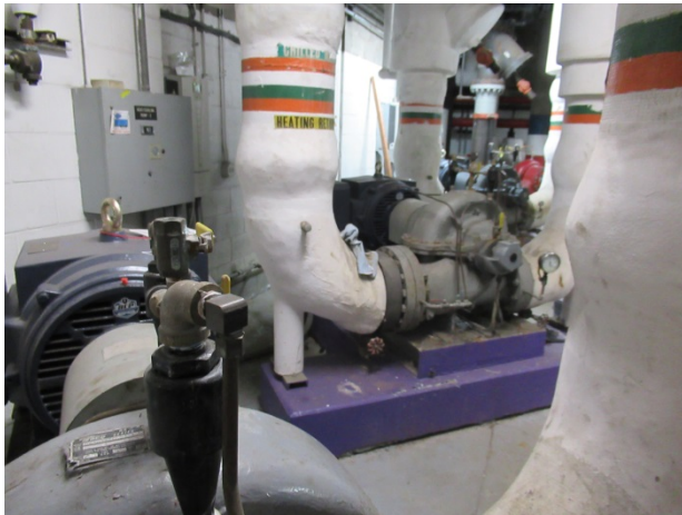
Dual temperature/fan coil loop pumps
