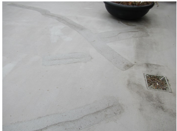
Crack repairs at waterproof coating at 2 nd floor concrete roof system
