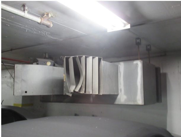
Original garage heater
