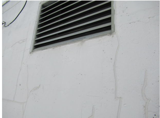
Repaired cracks at penthouse concrete
