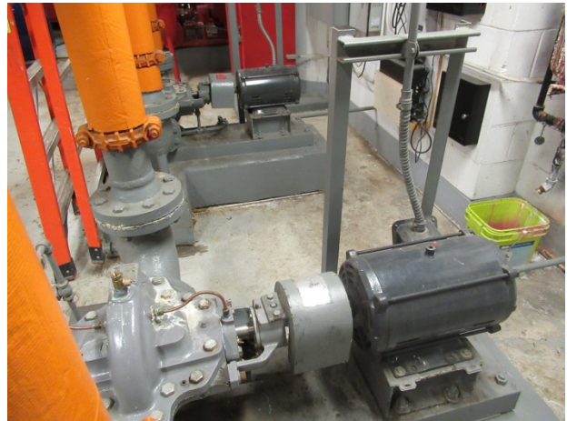
Pumps for fin tube radiators
