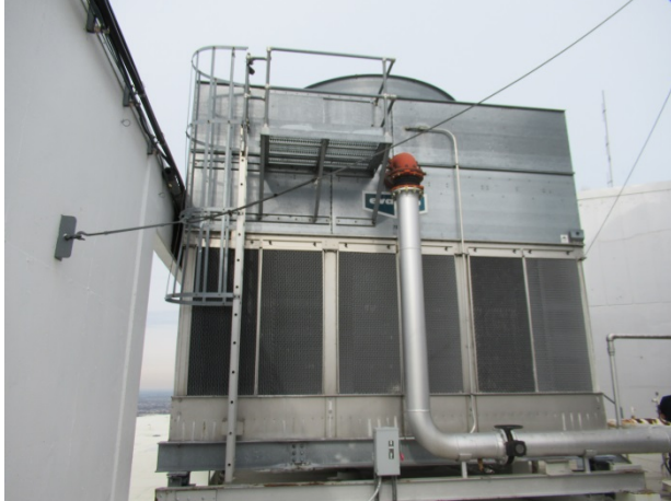
Residential unit cooling tower
