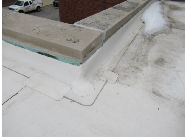
Roof system at perimeter at 2 nd floor northwest
