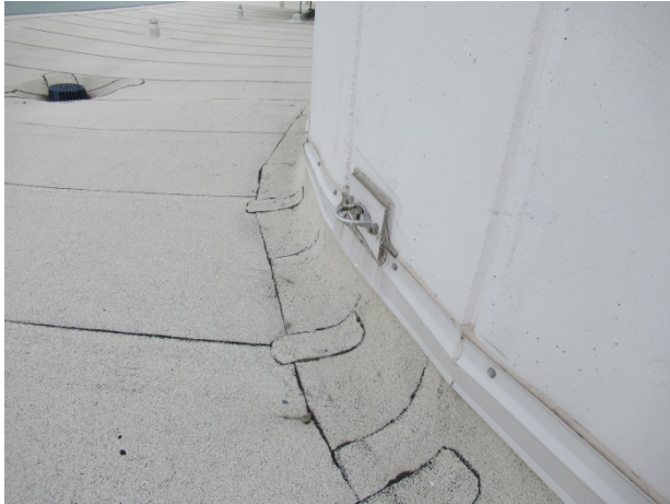
Main level roof system at perimeter termination
