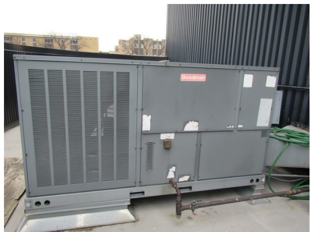
Racquetball court air handling unit
