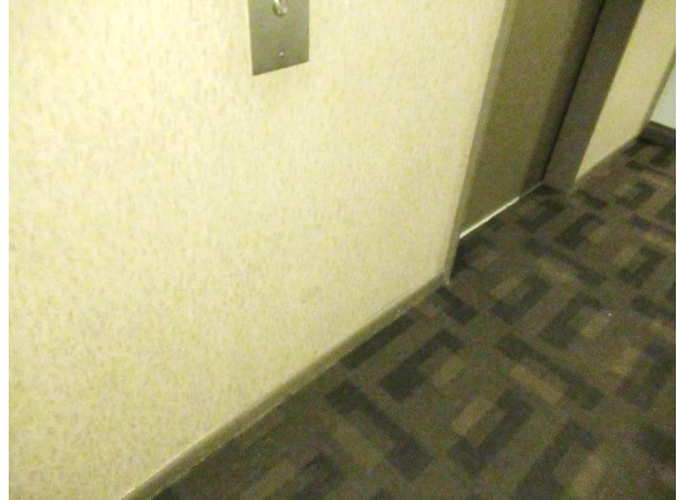
Typical damage at elevator foyer wall covering
