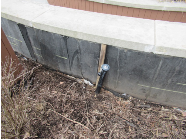
Recently replaced waterproofing system at 2 nd floor planter
