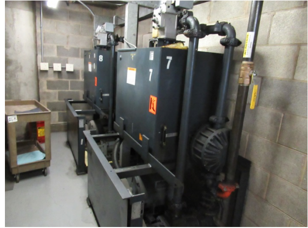
Power unit housings for the garage elevators
