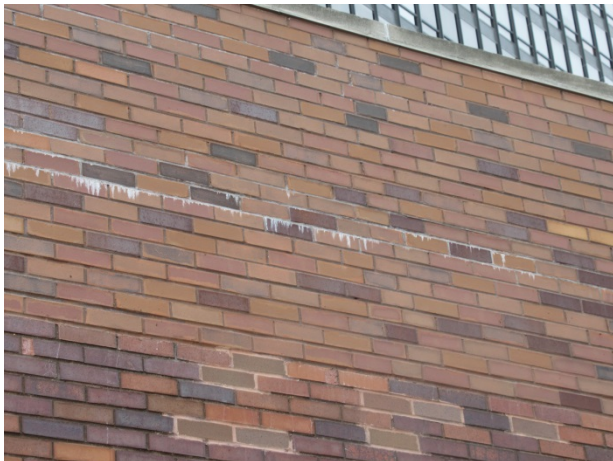
Evidence of water infiltration at masonry wall
