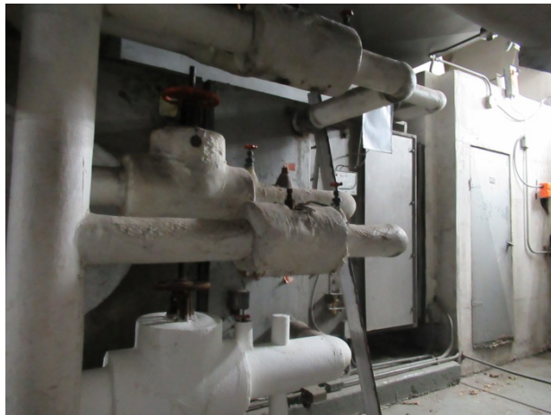
Lobby air handling unit
