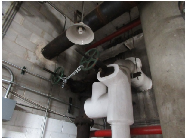
Valves at main water connection
