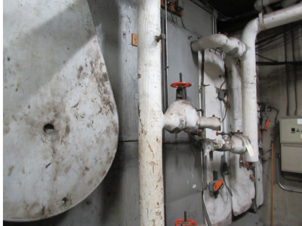
Corridor air handling unit
