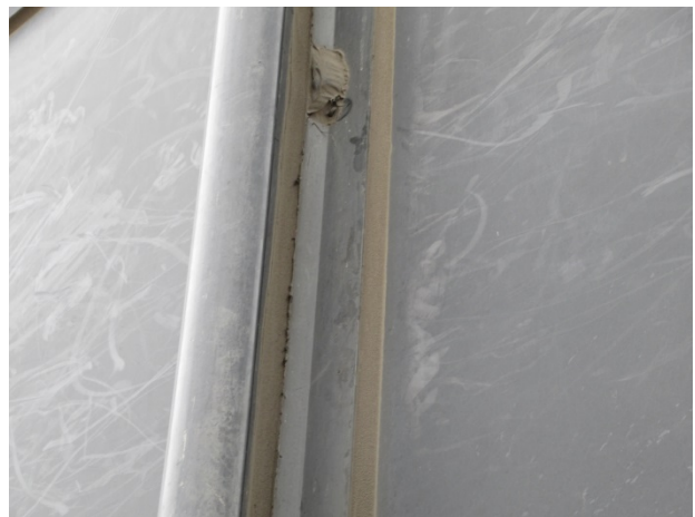
Sealant deterioration at metal/metal interface
