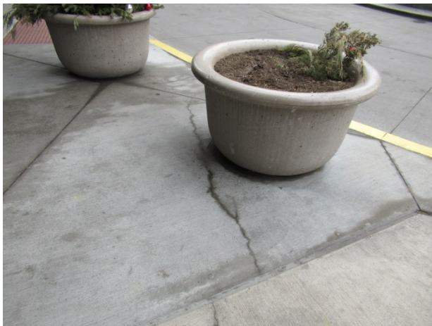
Crack in concrete at plaza
