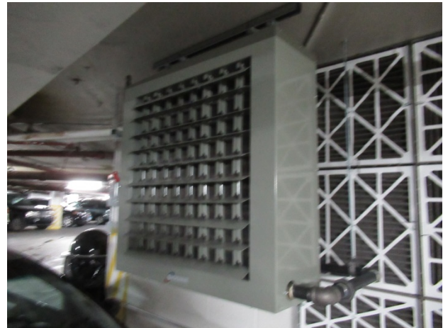
Recently installed unit heater
