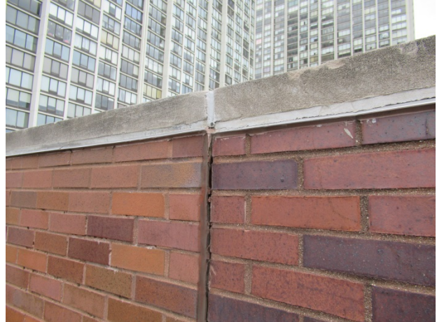
Masonry deflection at parapet wall
