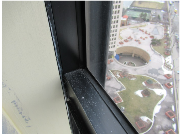
Residential unit curtain wall system at interior seals
