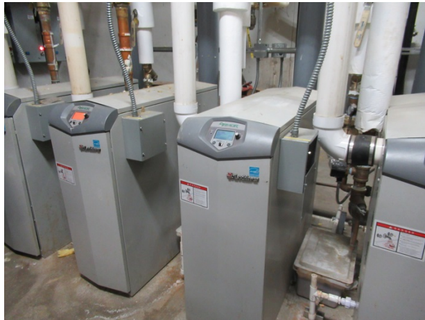
High zone domestic water boilers
