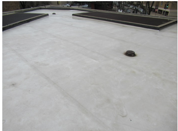
Roof system at 2 nd floor southwest
