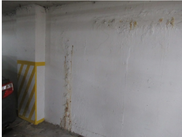
Seepage at garage lower level wall
