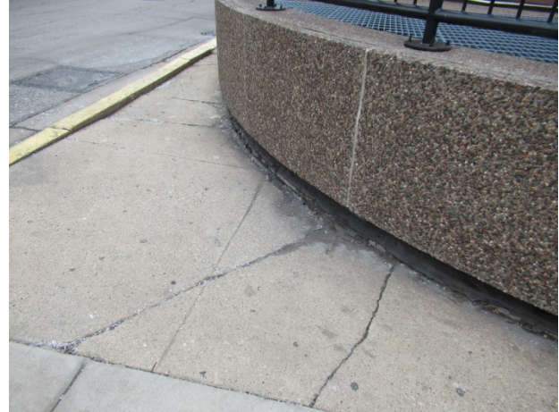
Concrete cracks
