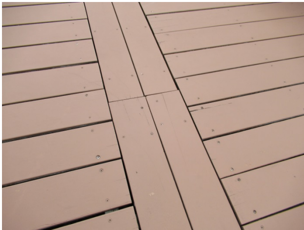
Weathered wood at 2 nd floor sun deck
