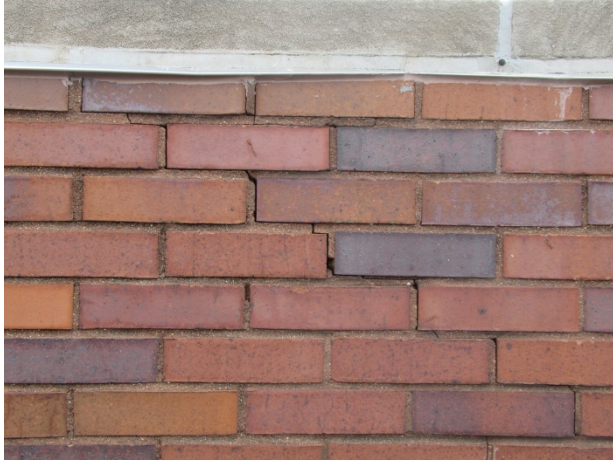
Masonry crack at parapet wall
