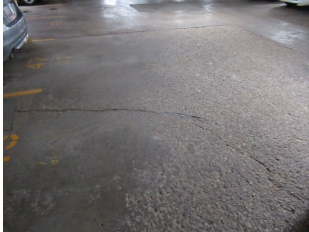
Concrete floor cracks and surface spall
