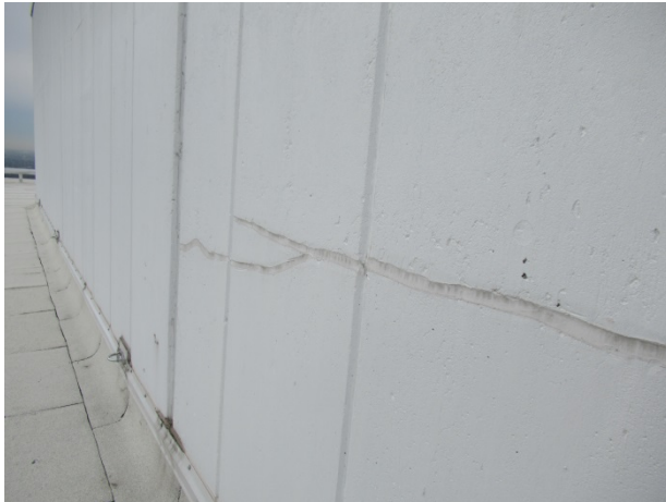
Repaired cracks at penthouse concrete
