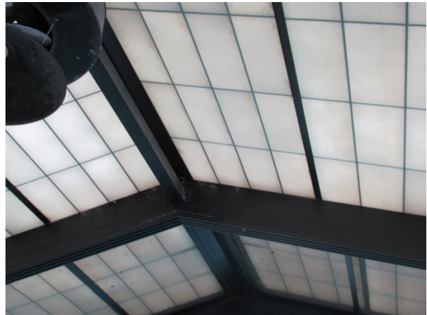
Evidence of water infiltration at pool enclosure
