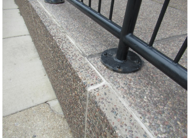
Sealants at plaza joints
