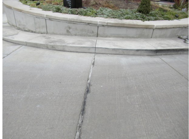
Sealant deterioration at circle driveway
