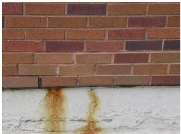
Evidence of water infiltration at masonry wall and lack of base flashing
