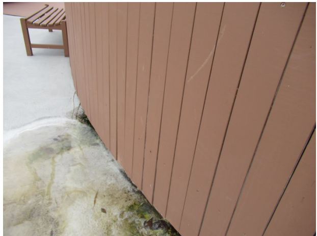
Wood at planter wall at 2 nd floor sun deck
