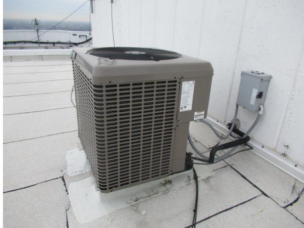
Condensing unit for elevator room
