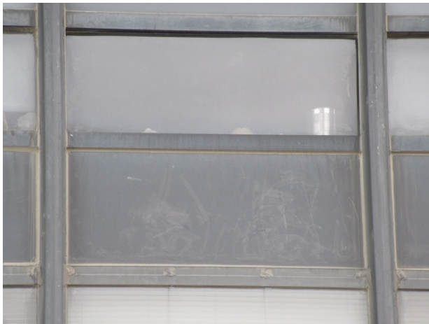
Spandrel panel dirt build-up
