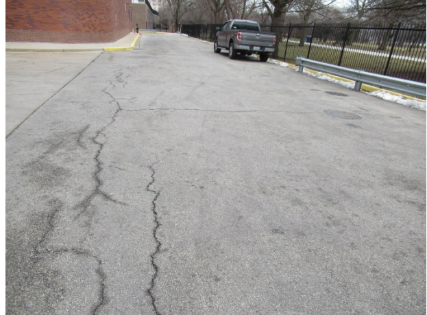
Pavement deterioration at east perimeter
