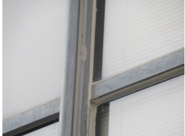
Sealant at metal/glass and metal/metal interfaces
