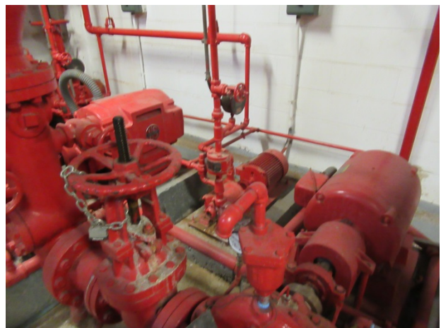
Fire suppression pumps
