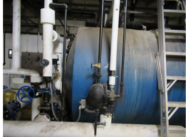
Boiler feed water system
