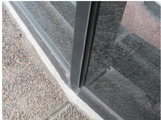
Lobby window system
