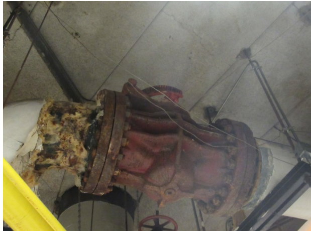
Valve to be replaced in near term
