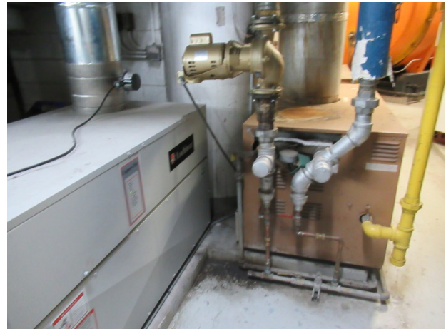
Low zone domestic water boilers
