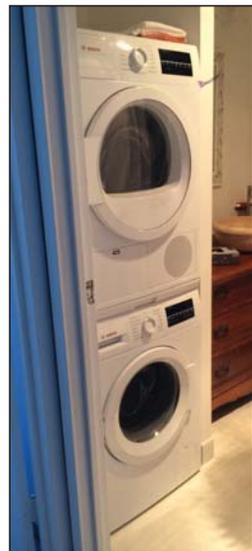
One more thing: By sacrificing the bathroom linens closet, Paula was able to install a Bosch washer and dryer. These are separate machines, better than a "combo," with the dryer on top. Note that 220 volt electric service was required in the bathroom, plus extensive plumbing.
