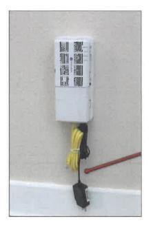
This outlet box, is just a bit bigger than a typical electric outlet. It does need to be plugged in, so ideally will be next to an outlet. Yhe red pointer shows where the fiber strand will come up from the base – and again, where it is painted over it is barely noticeable. This location would then be the hub to provide either
