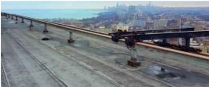
*see photo). But neither the bolts nor the railing is adequate for a building of our height, according to the new regulations.*
