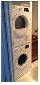
One more thing: By sacrificing the bathroom linens closet, Paula was able to install a Bosch washer and dryer. These are separate machines, better than a "combo," with the dryer on top. Note that 220 volt electric service was required in the bathroom, plus extensive plumbing.
