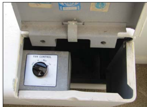
Top: A typical bedroom convector. Bottom Left: As example of a corroded drain pan from a leaking shutoff valve. Bottom Right: The all too familiar control knob that controls the motor speed of fan.
