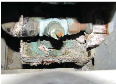
Top: A typical bedroom convector. Bottom Left: As example of a corroded drain pan from a leaking shutoff valve. Bottom Right: The all too familiar control knob that controls the motor speed of fan.
