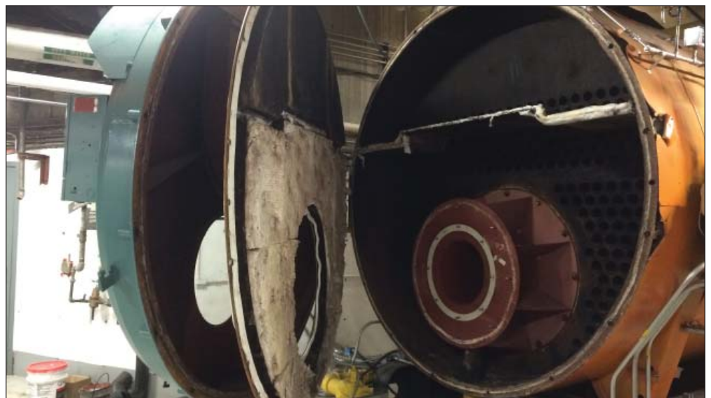
The boilers are opened during the summer months to perform regular maintenance.
