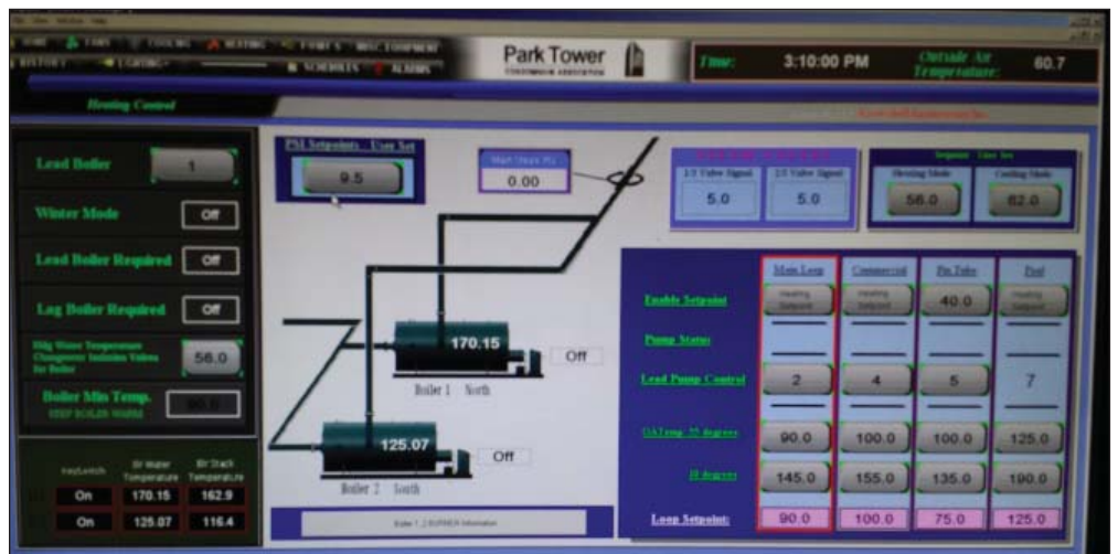
A view of the computerized control panel.
