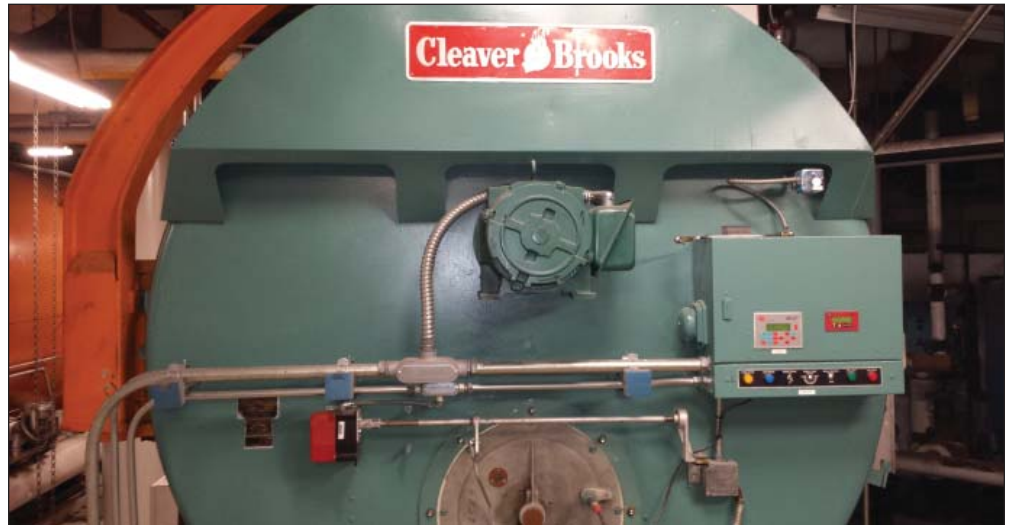
Above is the front door to one of Park Tower's two massive boilers.
