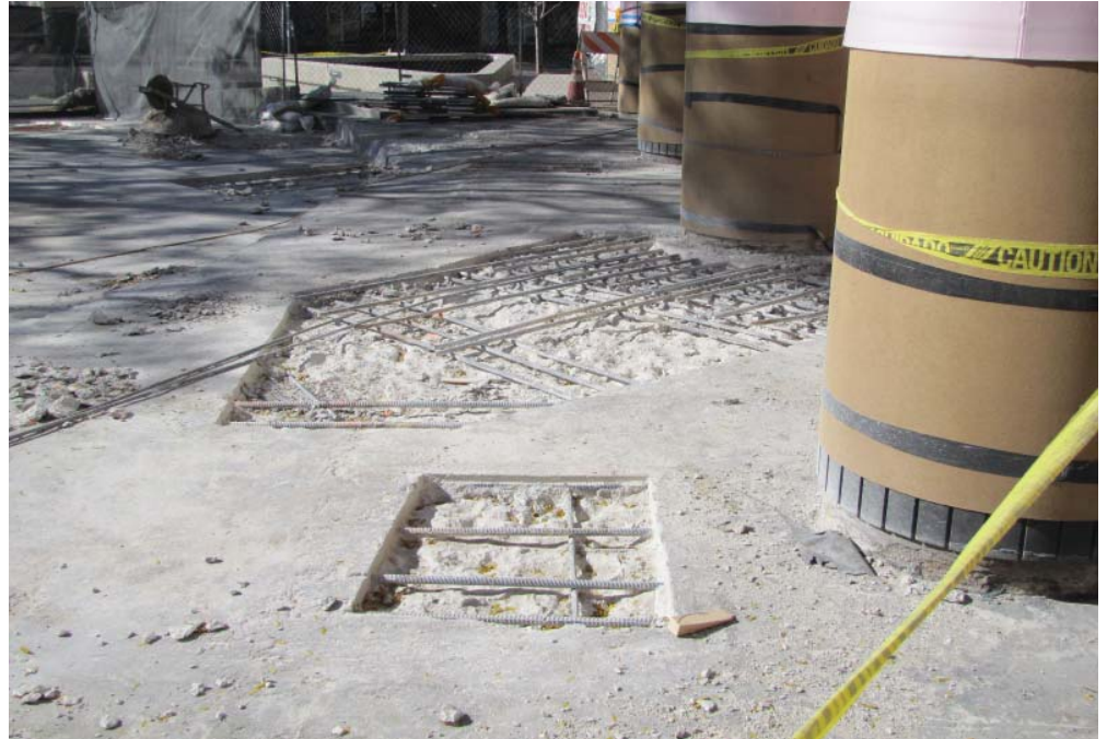
Repairs to the underlying concrete layer in the circle drive, where damaged concrete is removed, exposing the structural rebar.
